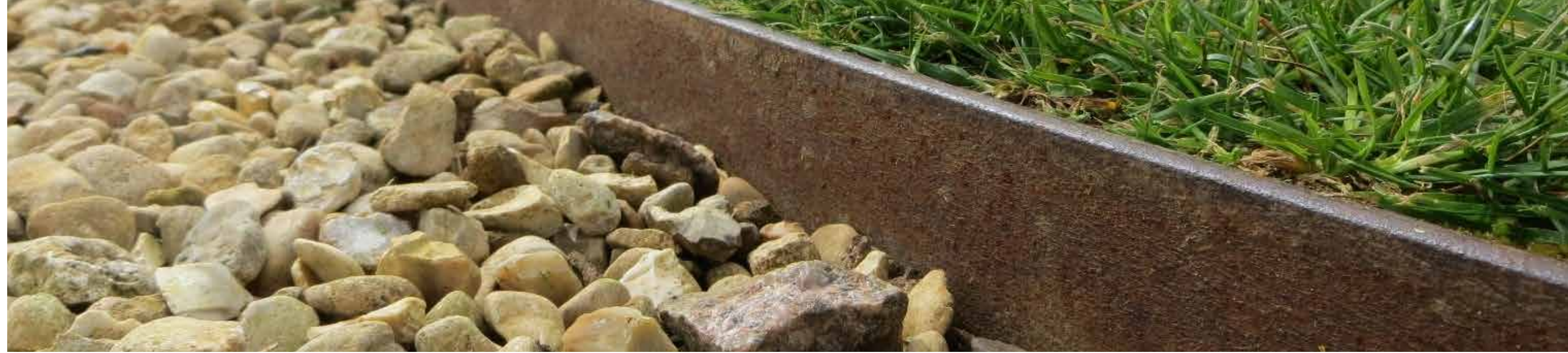
Steel edging restraint to retain gravel drive
